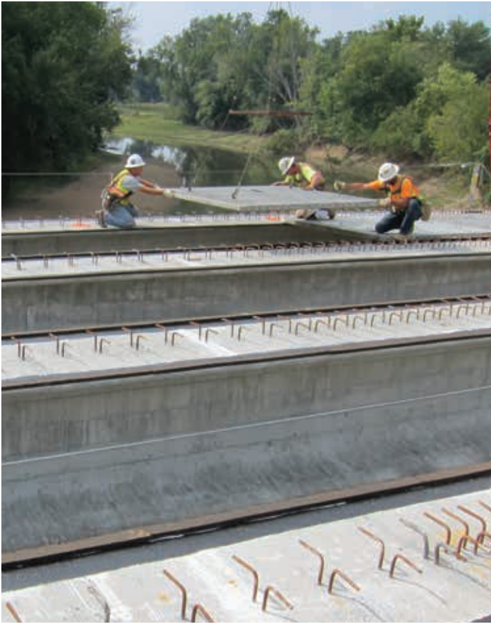
Above left: Workers place prestressed-precast concrete deck panels on a bridge near Jefferson City, Mo. Felt bearing pads like the one pictured above, right, are placed between concrete girders and deck panels to prevent cracking as the bridge moves during temperature changes. (Photos by Terry Barner)
